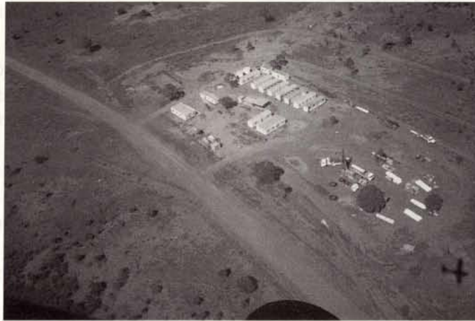
An aerial photo of remote exploration camp designed and supplied by Flexihire.
